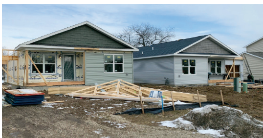
New home construction earlier this year on Kennedy Drive
