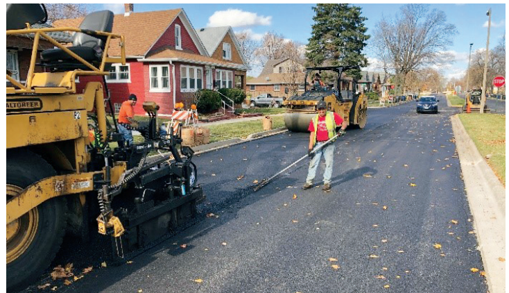
Roadway resurfacing on Adams Street
